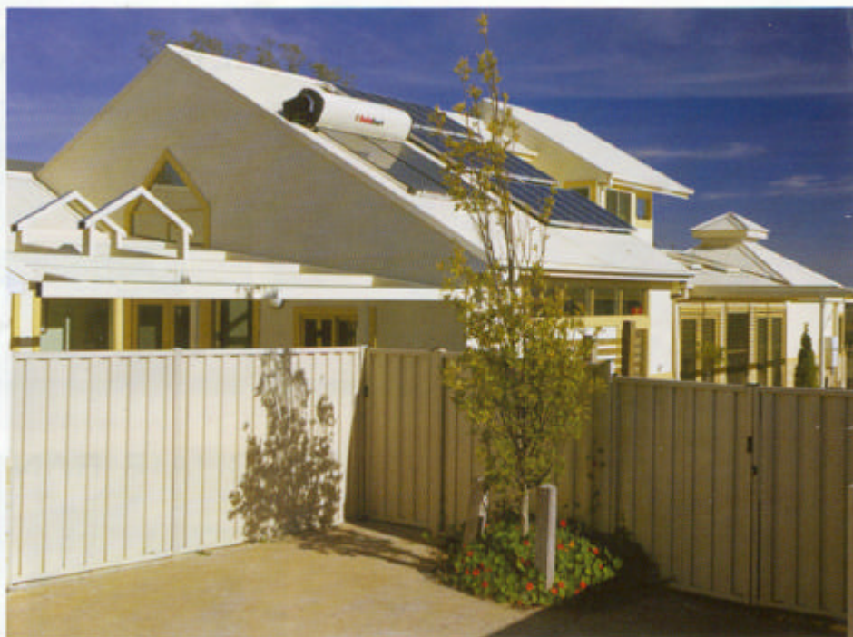
Light-coloured Colorbond® steel deflects sunlight to minimise heat entering through the roof in this energy-efficient building.
